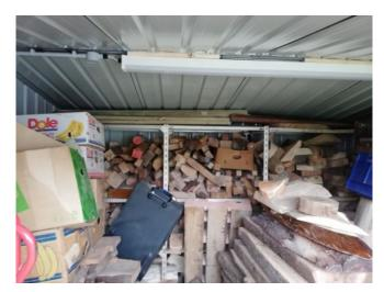
Any decent shed must have power and lighting but you cannot just run an extension cord out to the shed when needed. We had to make sure that you and anyone that might want to plant a tree were safe. External signs for the buried cables and internally, strip lighting, fuse box and power socket.
